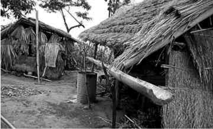
TYPICAL HOUSES. NOTE THE RAID WATER COLLECTION SYSTEM.
